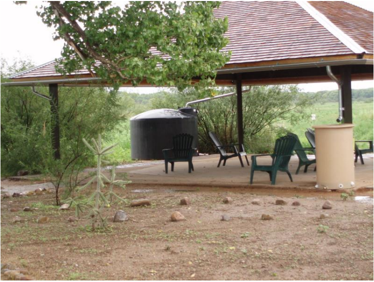
The amphitheater at the San Pedro House with its new rain gutters and water storage containers Photo by Ted Mouras
