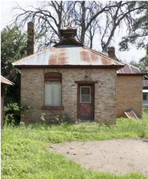
Boquillas Ranch Headquarters. Photo by Ron Stewart
